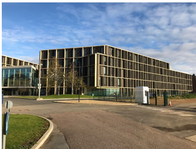
数学科の建物 (Andrew Wiles Building)
