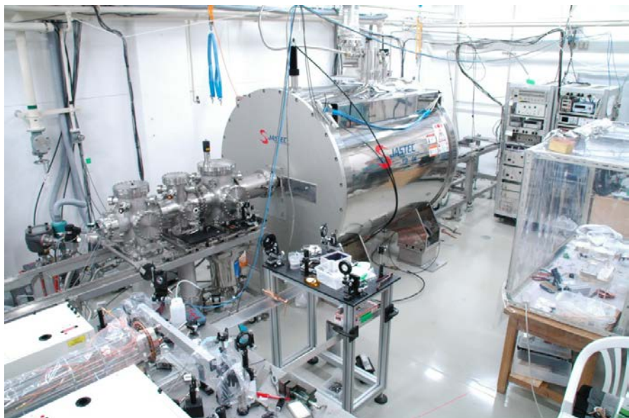
Magnet is 1.85 m in length and 2.2 m in height
